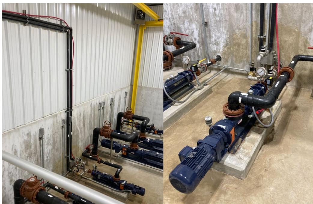
Figure 73. Polymer line (red) to CL2 HPC pump.
