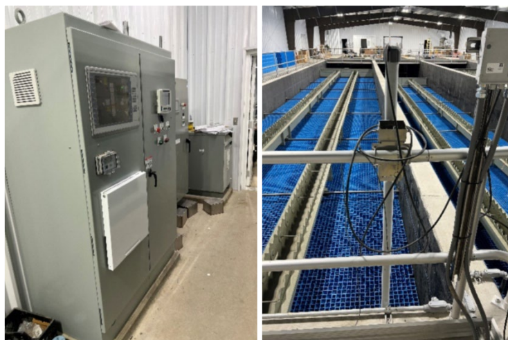
Figure 9. (left) Control panels for WVDEP's treatment monitoring, and (right) First and second clarifiers on standby for shakedown testing.
