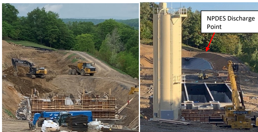
Figure 7. Early construction of the A-34 site (formerly lower ponds). Construction utilized preexisting pond to pour concrete forms.
